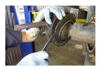
Using a standard screwdriver, remove the (2) retainer ring halves and knuckle ball seal.
